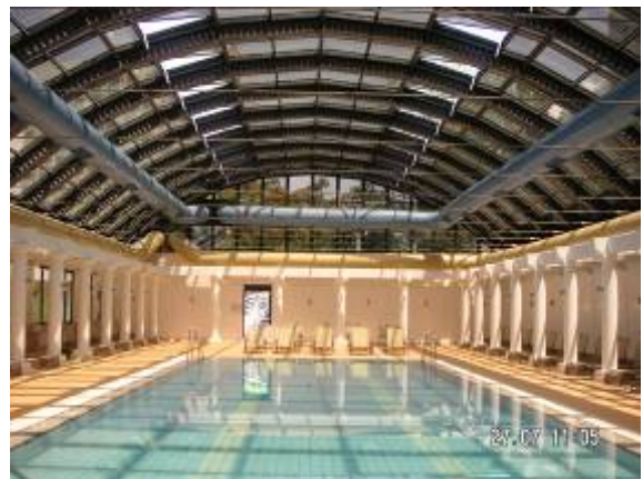
Swimming Pool Roof
