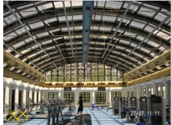
Fitness Centre Roof
