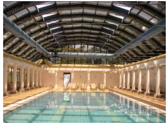
Swimming Pool Roof
